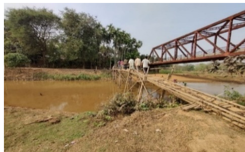
Villagers crossing the river through a temporary bamboo footbridge structure.
