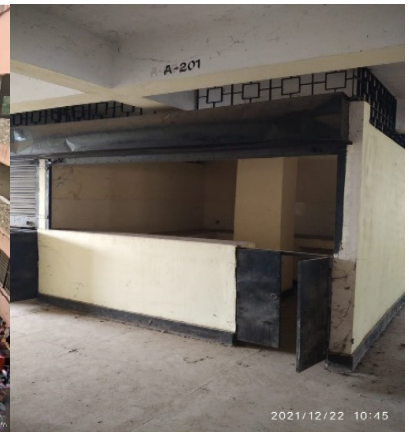
Photo-2: Stalls of Ampati market building lying unutilised.
