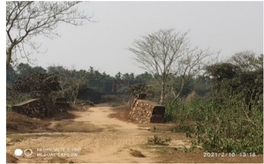
Photo showing non-existence of road formation.
